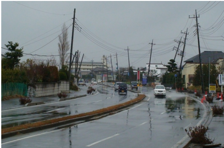
(a) Tilting and subsiding utility poles
