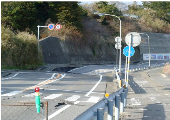
(b) Road near Nakaminato port
