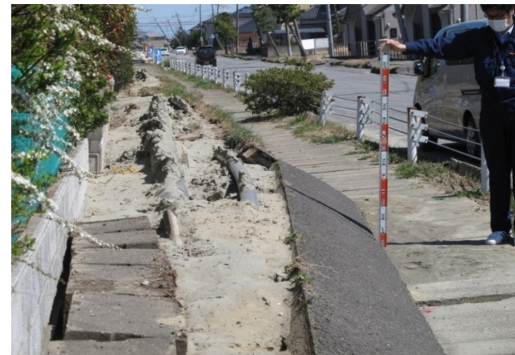
(b) Surfacing drainage tube (about 0.4m)
