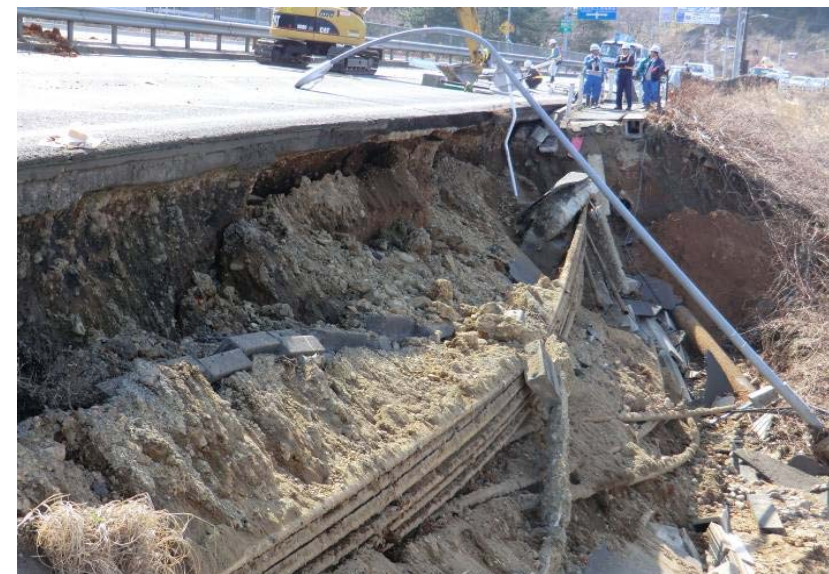
Damage of NTT' junction cable
