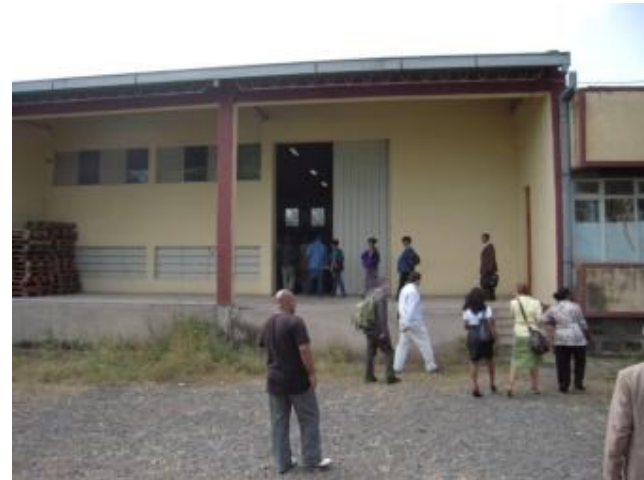
Demanufacturing Facility (DMF) located next to CRTC
