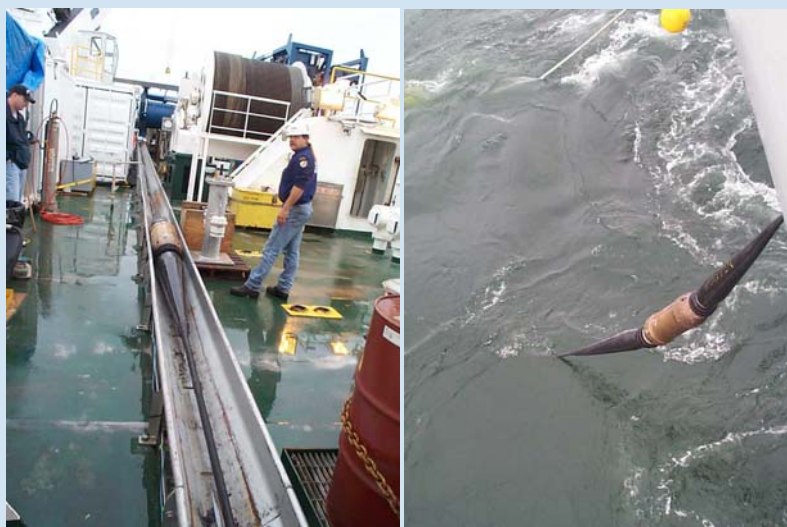
Figure 5: Optical repeaters are shown during a cable installation. System electronics and lasers are located in the copper-hued housing.
