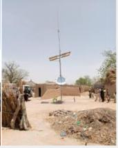
Remote AMN small site deployments that typically service populations of around 1 000 people. Coverage areas range from 1.5 to 3 km for the 12-m tower, and 3.5 to 7 km for the 20-m tower, depending on terrain.
