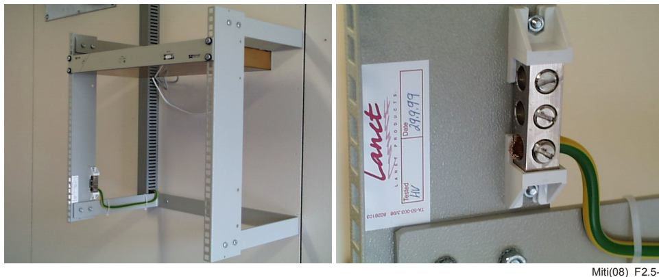
Figure 2.5-1 – System configuration (An example of mistakes in bonding)
