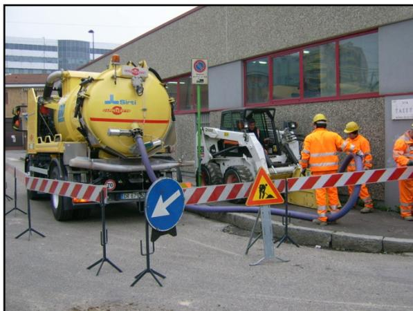
**Figure I.1 – Trench saw combined with suction machine**
