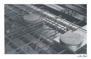
Figure II.8/L.59 – Example of cellular raceway installation
