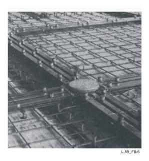
Figure II.6/L.59 – Example of under-floor duct installation
