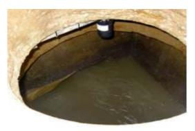
Figure 18 – SmartScan 50 non-contact gauging device equipped with sensors
