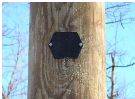
Figure I.2 – Tag installation
