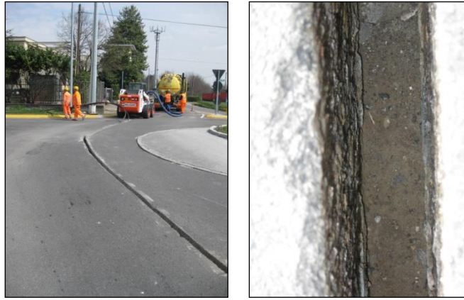
Figure I.2 – Cleaning of the site and inside the trench
