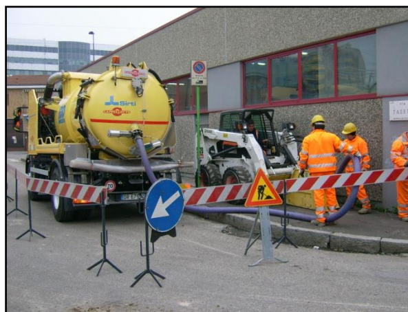
Figure I.1 – Trench saw combined with suction machine
