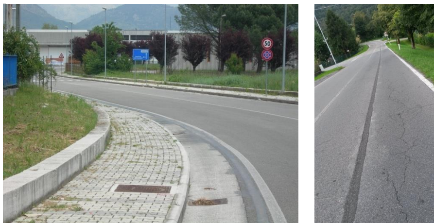
Figure 3 – Examples of micro-trench positioning
