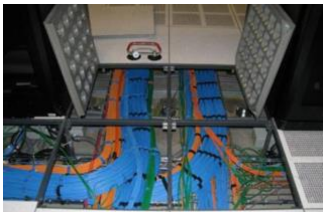
Figure 10 – Under floor cable runs
