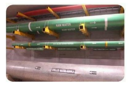
Figure 13 – Utility tunnel, showing waste and water pipes Source: [b-Gujarat]
