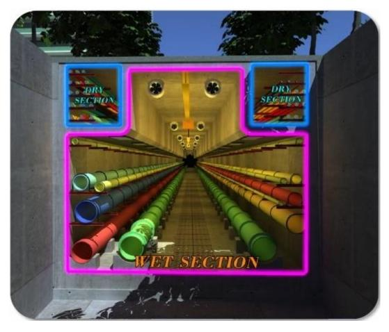
**Figure 10 – Utility tunnel, showing wet and dry sections** Source: [b-Gujarat]
