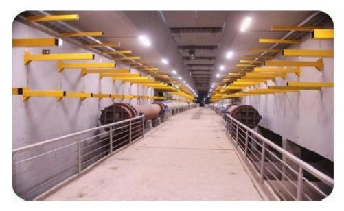
**Figure 12 – Utility tunnel, showing support brackets** Source: [b-Gujarat]
