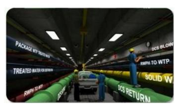
Figure 14 – Utility tunnel, showing district cooling system solid waste and water pipes Source: [b-Gujarat]
