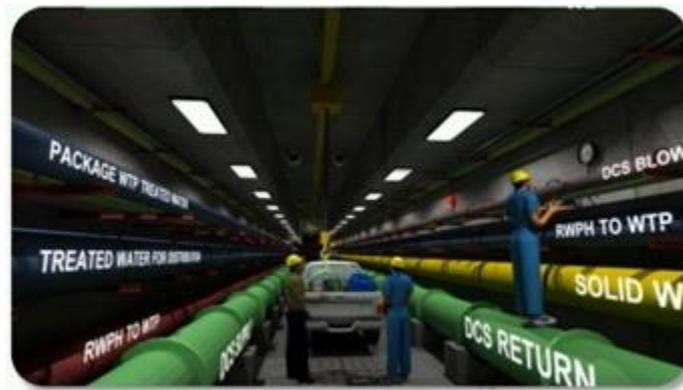
**Figure 14 – Utility tunnel, showing district cooling system solid waste and water pipes**
