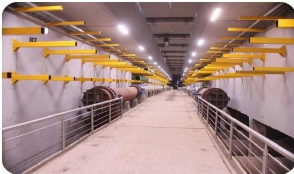
**Figure 12 – Utility tunnel, showing support brackets**
