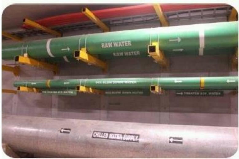
**Figure 13 – Utility tunnel, showing waste and water pipes**
