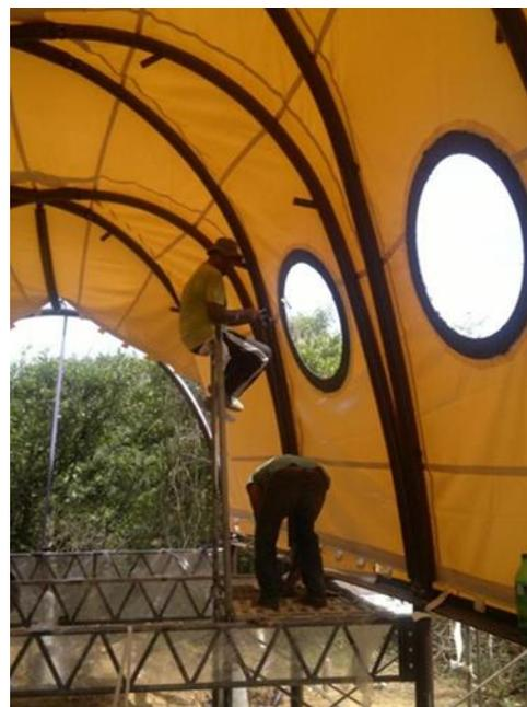
**Figure 13 – Membrane installation**
