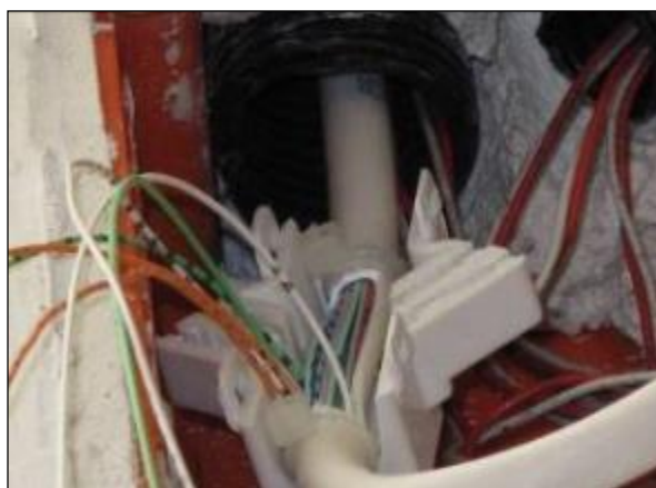
Figure II.6 – A window is open on the cable sheath
