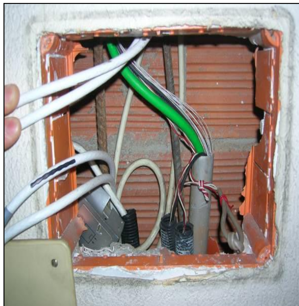
Figure II.5 – Riser cable installed in existing infrastructure
