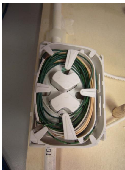
Figure II.7 – Installation of the fibre protection shell (left – different dimensions are available) with protection tubes or splice box (right)
