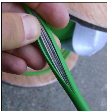
Figure II.6 – A window is open on the cable sheath
