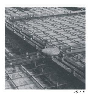
Figure II.6 – Example of under-floor duct installation
