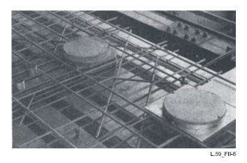
Figure II.8 – Example of cellular raceway installation
