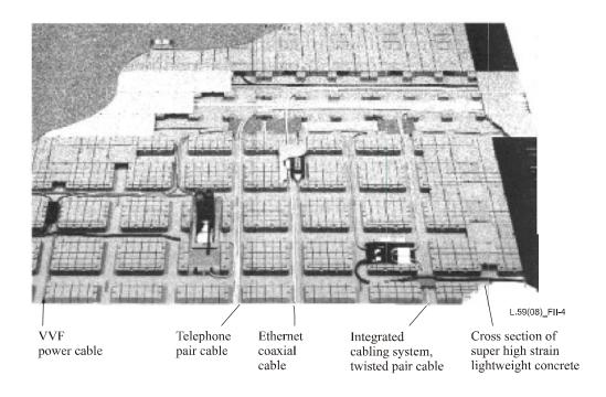
Figure II.4 – Example of simplified access floor system (floor-mounted type)
