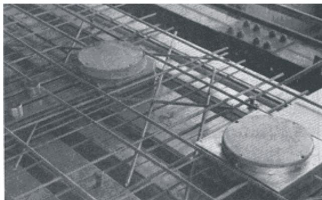
**Figure II.8/L.59 – Example of cellular raceway installation**
