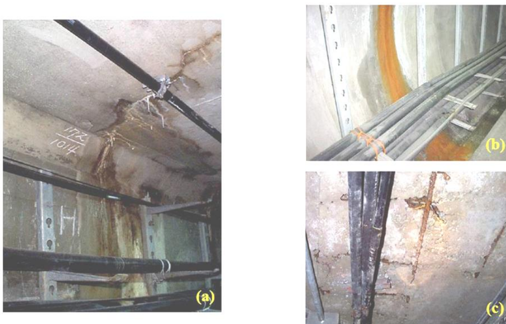
Figure I.1 – Typical types of deterioration: (a) cracks; (b) water leakage; and (c) corrosion of rebar
