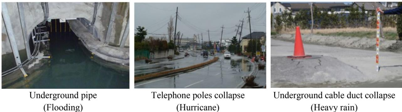
**Figure 1 – Examples of damage to electrical facilities due to climate change risk factors**
