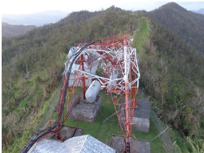
**Figure 3 –Telecommunication tower brought down by a cyclone [b-ITU-APRD]**
