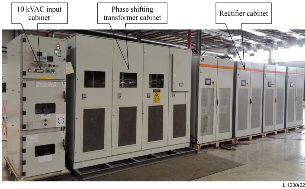
Figure I.1 – 10 kVAC input and up to 400 VDC output integrated power system testing
