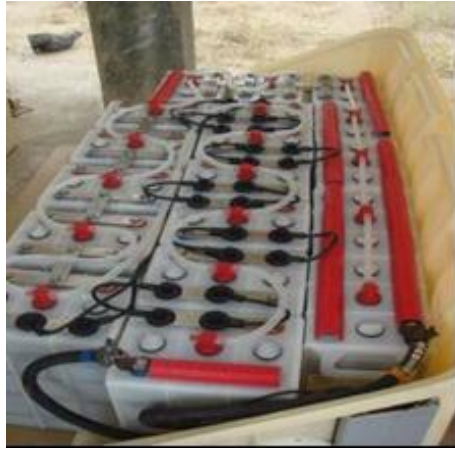
Figure I.7 – Example of a SAFT Sunica™ NiCd battery in an African country (courtesy of Orange)
