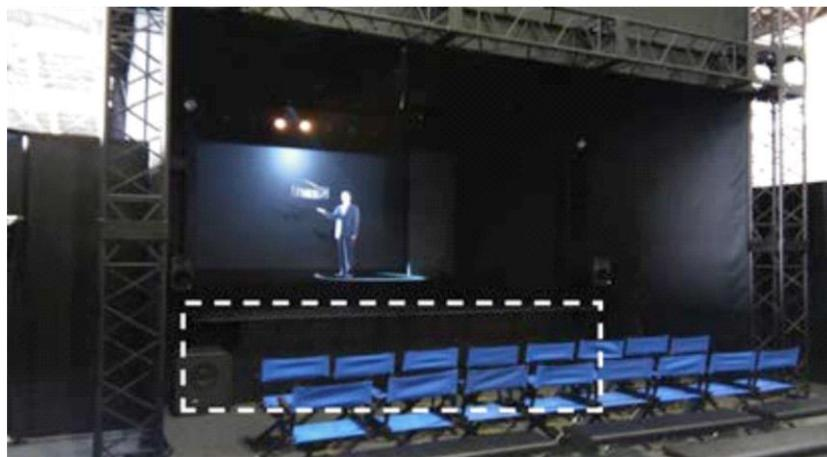
Figure I.2 – Front array embedded at the bottom of the stage (box with dotted line)
