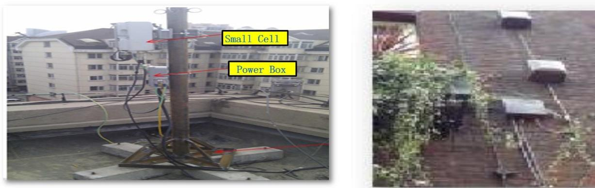
**Figure 7 – Schematic diagram of small cell installation**
