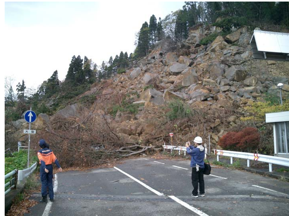
(Example of the site of a soil landslide)
