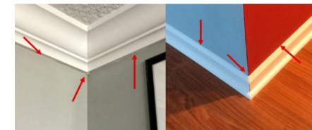
a) For method A - Installed 900 µm tight buffered fibre with adhesive
