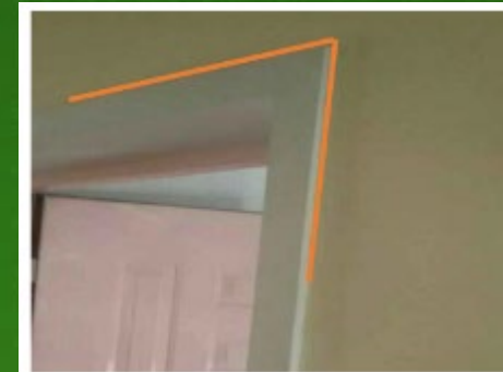
Installation of the in-home cable (indicated by orange line)
