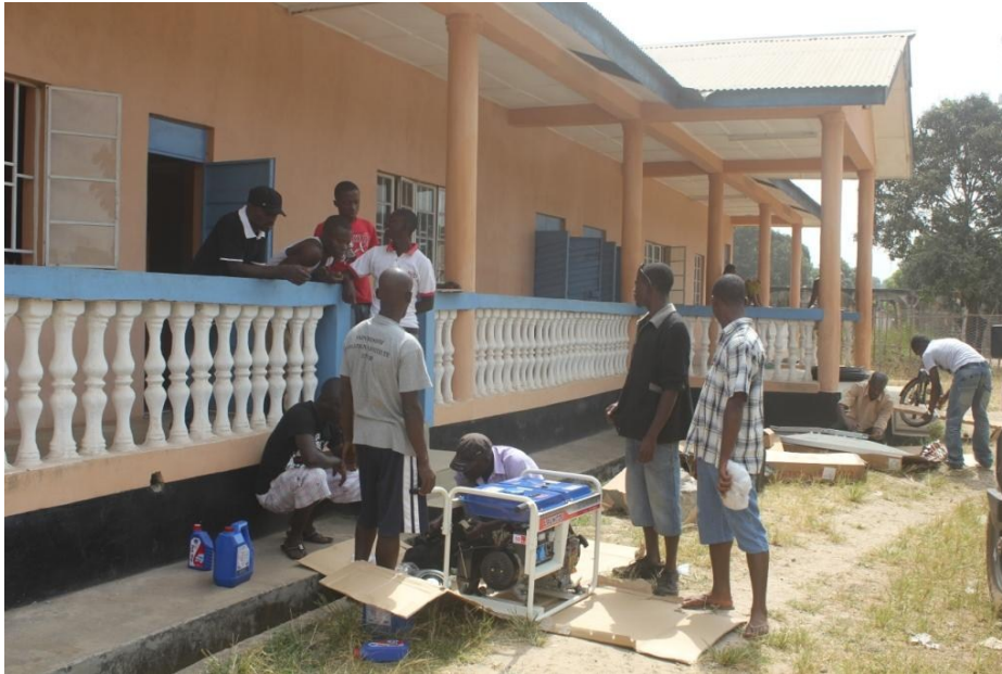
Picture 3: Installation Works at the Newly Constructed Mile 91 District Council Head Quarters
