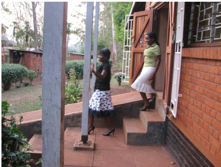
Picture 4- Newly Constructed ramp at the Mulanje MCT
