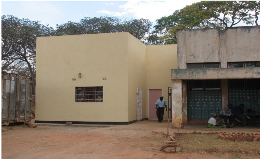
Picture 3 MACRA's Newly Constructed Building at Mchinji MPC
