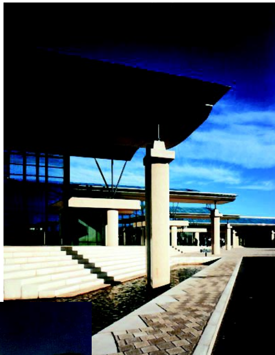
A view of the Cable & Wireless campus (ITU 000057)
