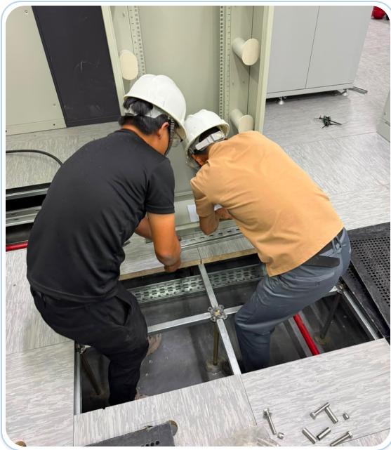
Cable Landing Station
