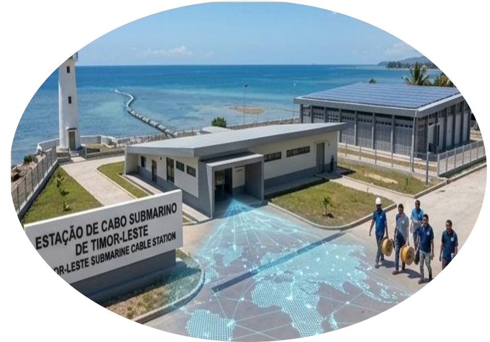
Timor-Leste Submarine Cable Station
