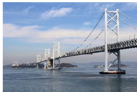
Tension monitoring for cable-stayed bridge
