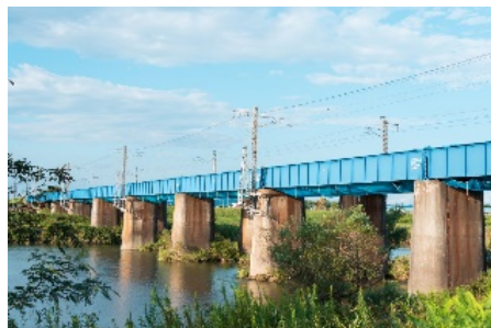
Bridge pier monitoring
