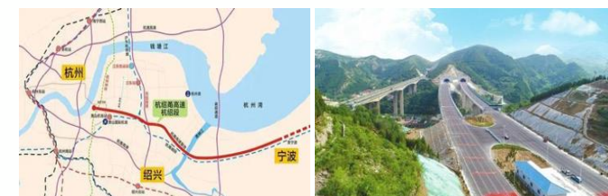
Hangshaoyong Smart Expressway
