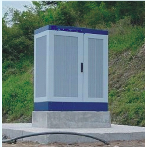
Figure 4-18: Example of cabinet for broadband services
