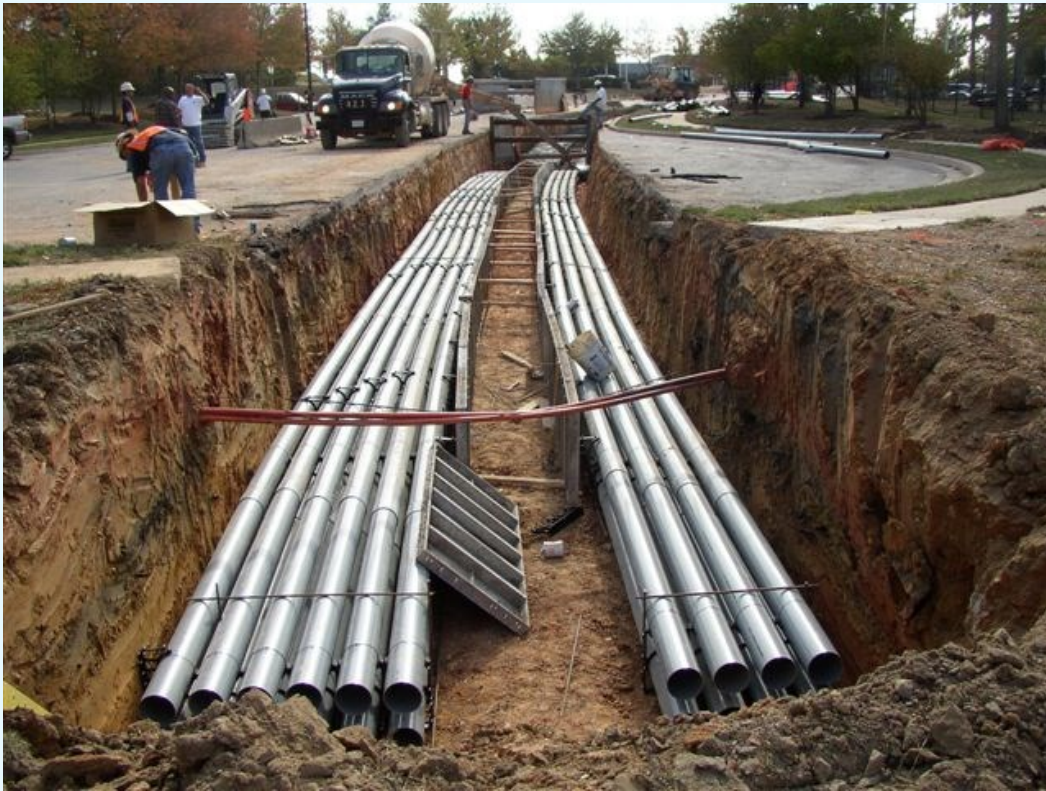
Figure 4-11: Ducts laid in a trench
