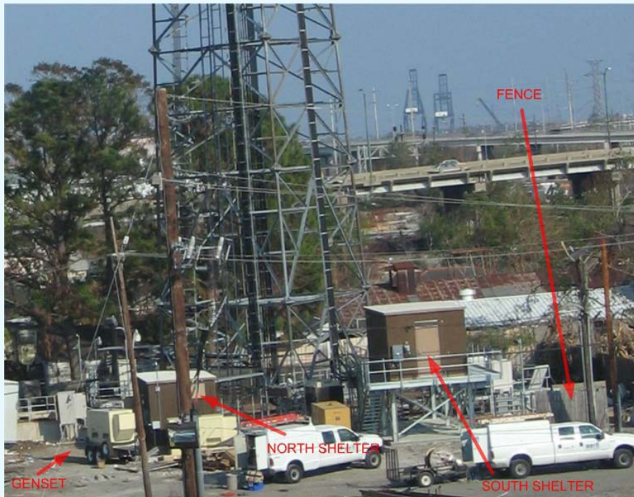
Figure 3-17: Cell site in New Orleans with 2 indoor and 2 outdoor base stations. The south shelter is on the front of the picture
