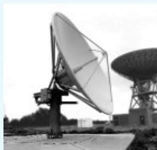
Figure 2-16: Basement and antenna of a satellite system
