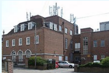
Figure 5-5: Cell site placed atop an existing building
