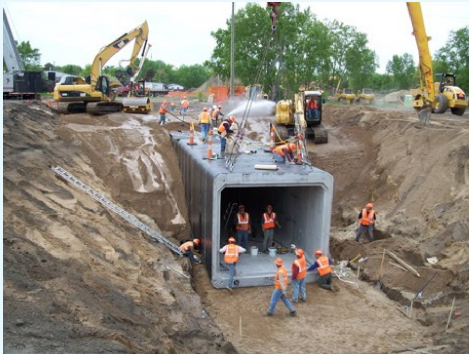
Figure 4-12: Open-cut tunnel
