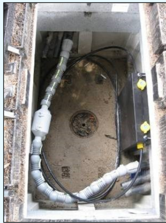
Figure 4-20: Protection system for extra length cable in handholes
