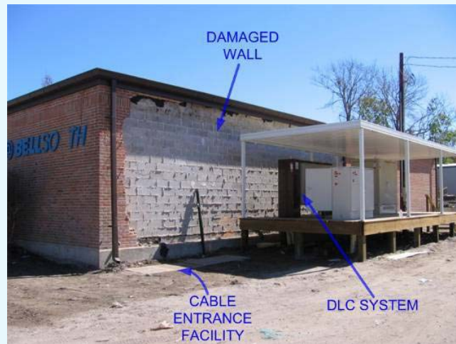
Figure 3-14: Pass Christian CO showing the DLC system used to replace the destroyed switch
