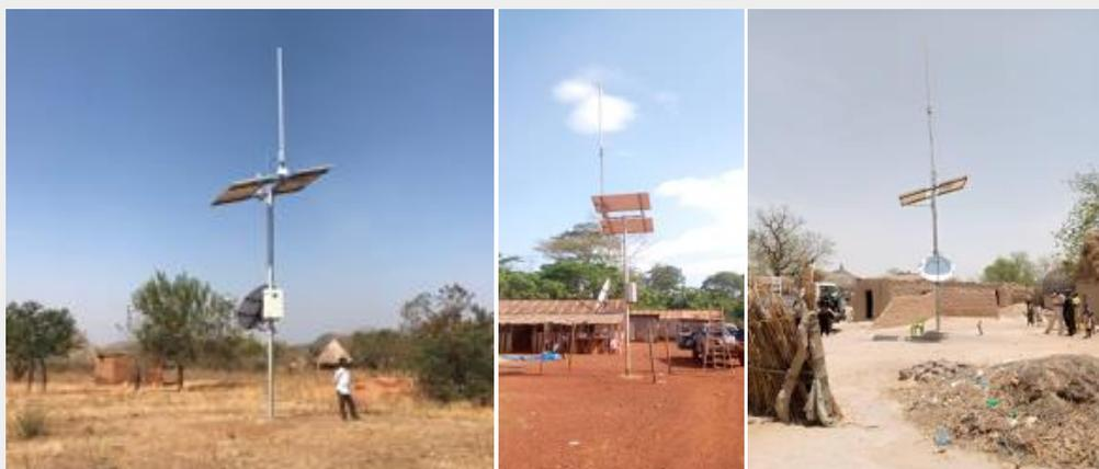
Remote AMN small site deployments that typically service populations of around 1 000 people. Coverage areas range from 1.5 to 3 km for the 12-m tower, and 3.5 to 7 km for the 20-m tower, depending on terrain.
