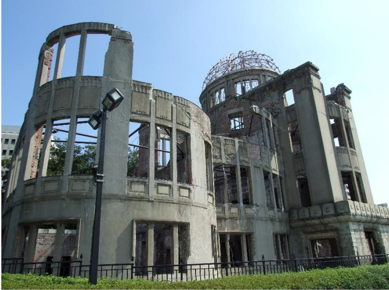
The "A-bomb Dome" was originally constructed as the Hiroshima Prefectural Commercial Exhibition on the eastern riverside of the Motoyasu-bashi Bridge in 1915. This facility was a three-storey (partly steel-structured) brick building designed by a Czech architect, Jan Letzel. The centre of the facility is the five-storey staircase structure, on which a copper elliptical dome is positioned.
