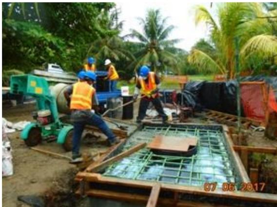
Concrete Pouring of BMH top slab
