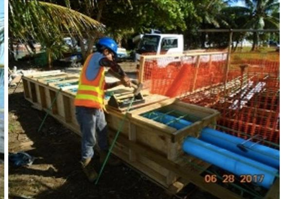
Installation of PVC 2 ea. 6" C-900 pipes, formworks and bracing for the 1st Pre-cast of the Seaward Duct
