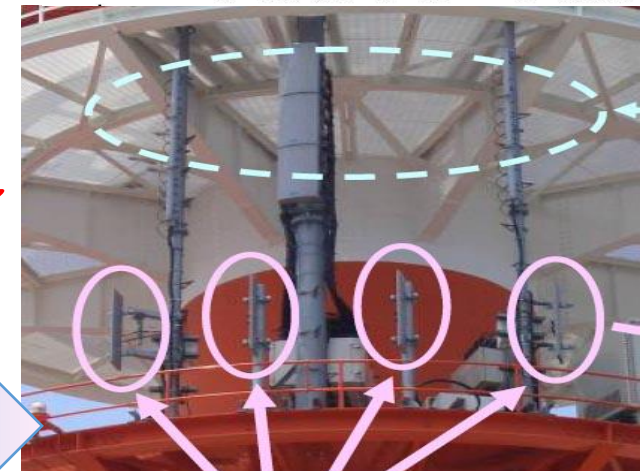
Large antenna spacing ( >10\lambda ) : suitable for SDM
