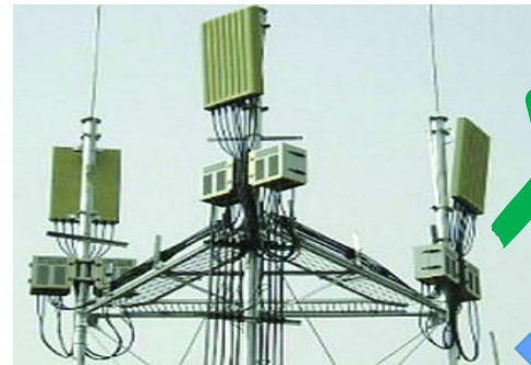
Small antenna spacing ( \lambda/2 ) : Suitable for beam forming
