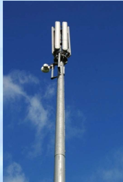
(Passive) Mast Sharing and (Active) Mast and Antenna Sharing
