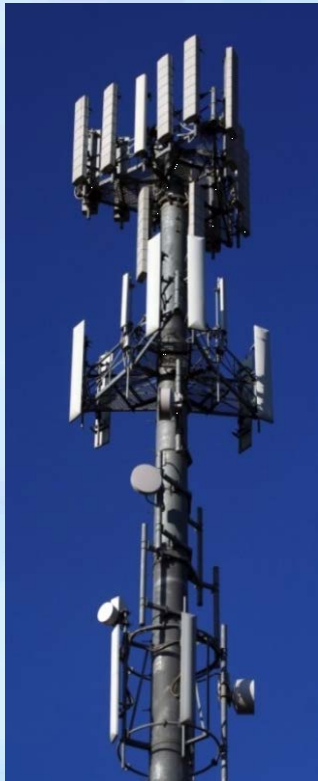
(Passive) Mast Sharing and (Active) Mast and Antenna Sharing
