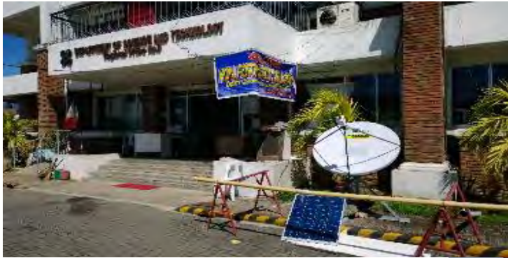
DOST Region 8 Office (showing solar-powered VSAT) where the base station was located
