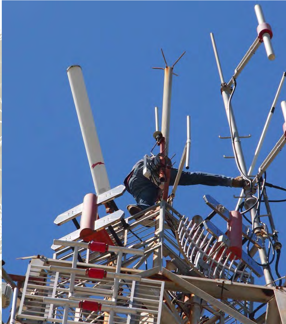
Working to straighten an antenna at the top of the mast with no safety gear.
