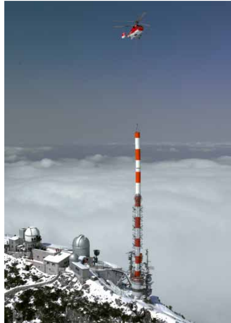
DAB+ / DVB-T antenna being installed on the Wendelstein mountain.
