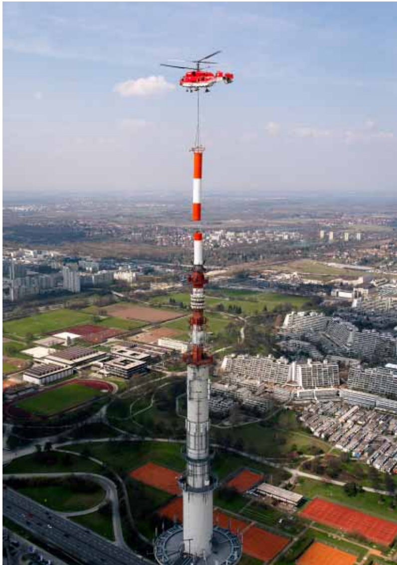
DVB-T antenna being installed on top of the „Olympiaturm“ television tower in Munich.
