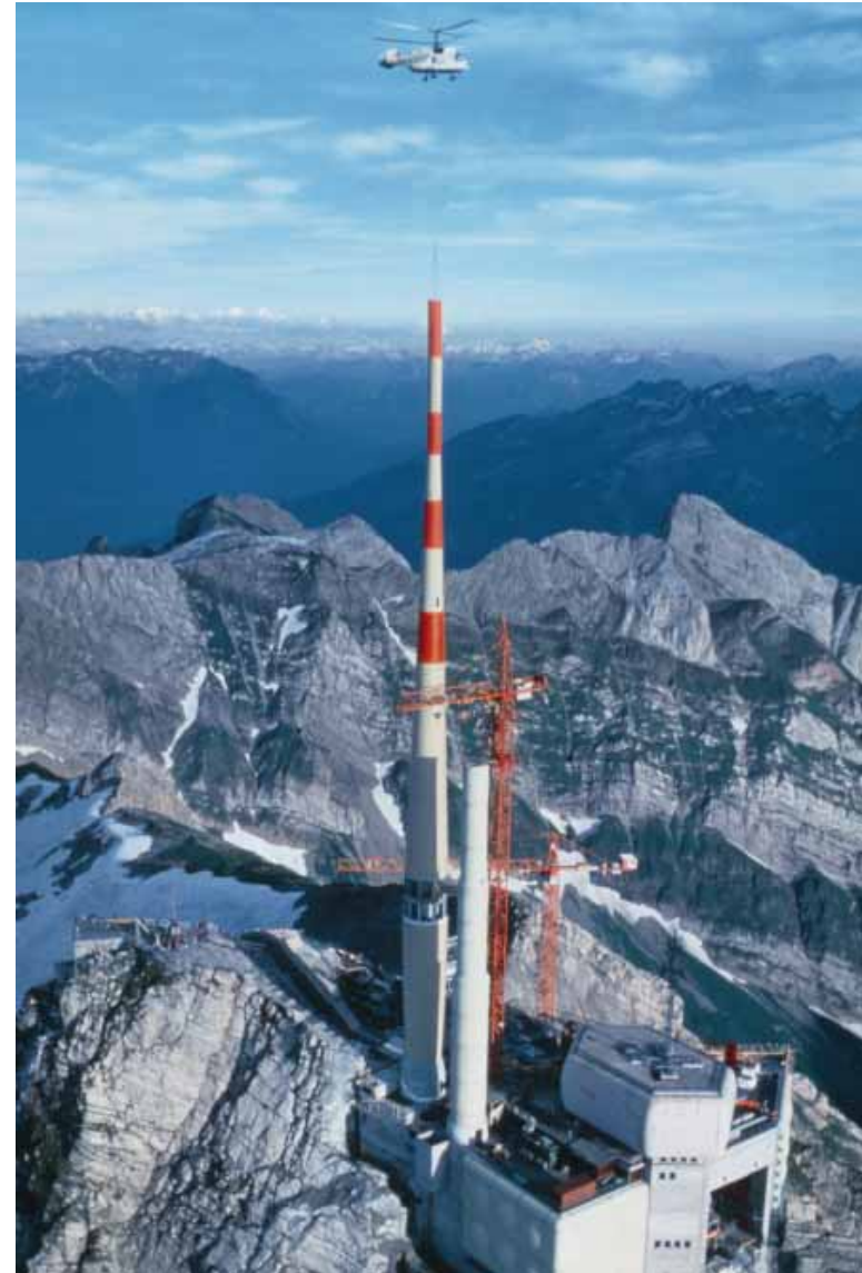
Kathrein antennas on Mount Säntis, Switzerland
