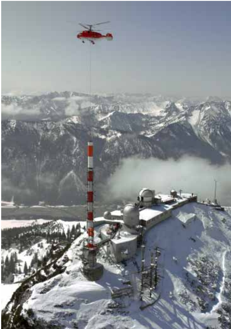
DAB+ / DVB-T antenna being installed on the Wendelstein mountain.
