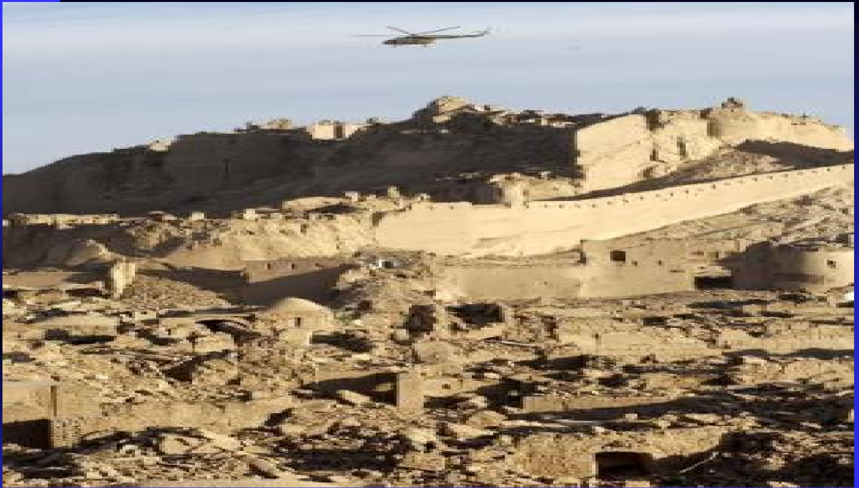
Citadel after the earthquake
