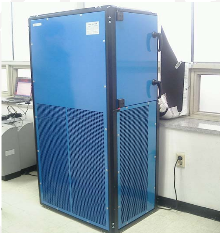
Indoor winter electricity-saving device in base station
