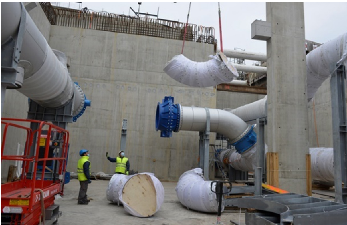
Figure 5: Installing the GeniLac pipelines
