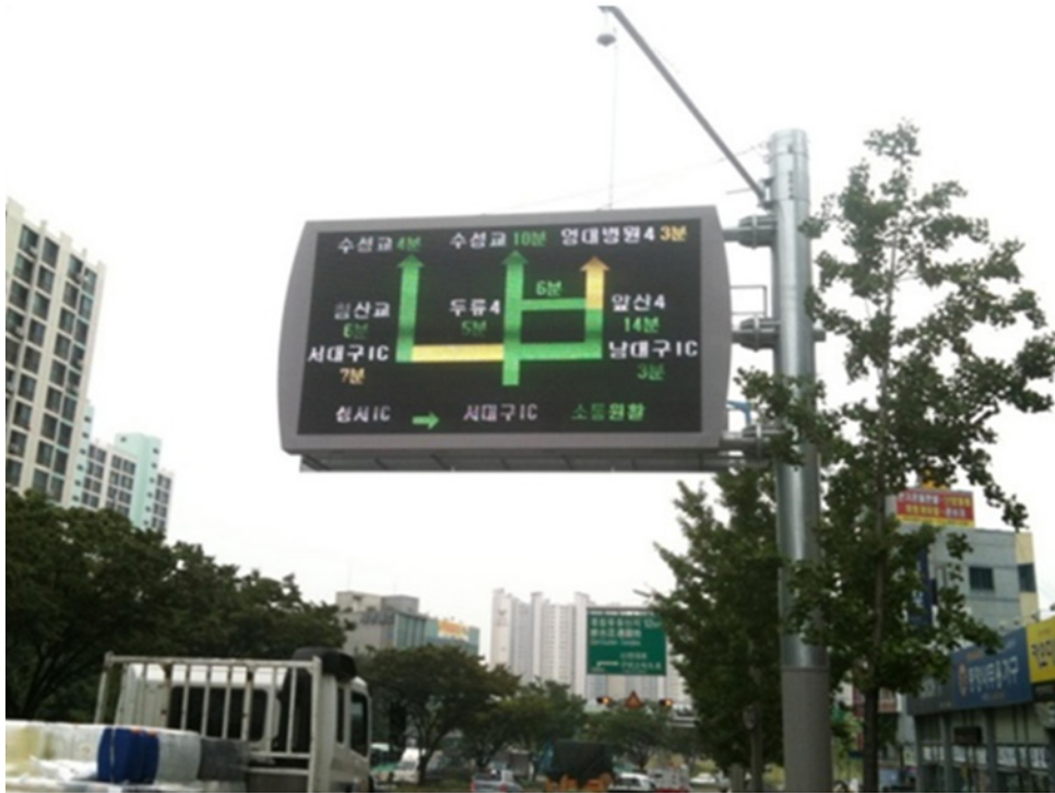
Figure 14: Traffic variable message sign
