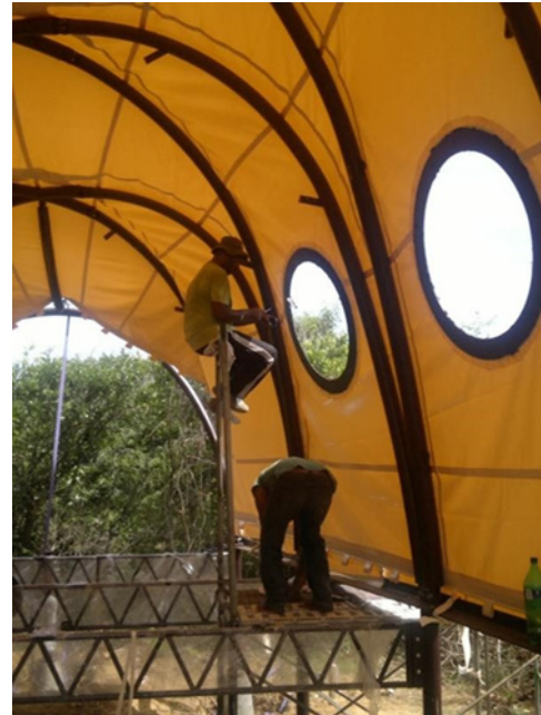
Figure 5: Membrane installation
