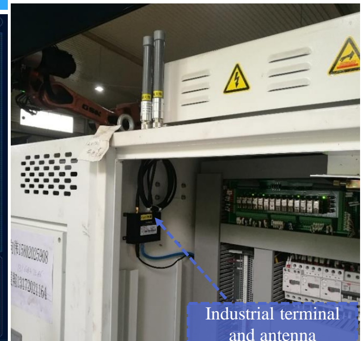
Industrial center access equipment and antenna
