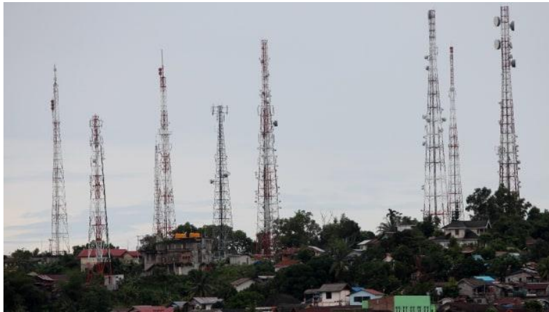
FIGURE A3-1 Microwave Link Towers in Indonesia
