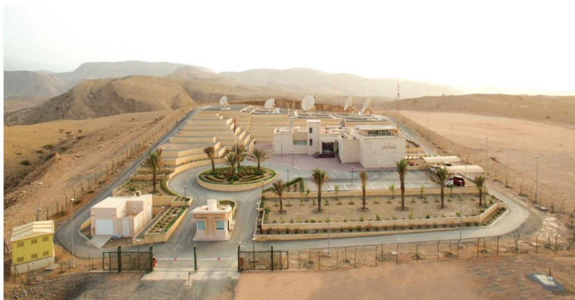
FIGURE 28 Site de la station SRMS
