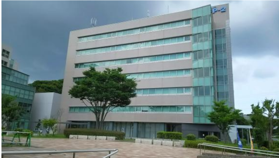
Snapshot of the light gauge steel building
