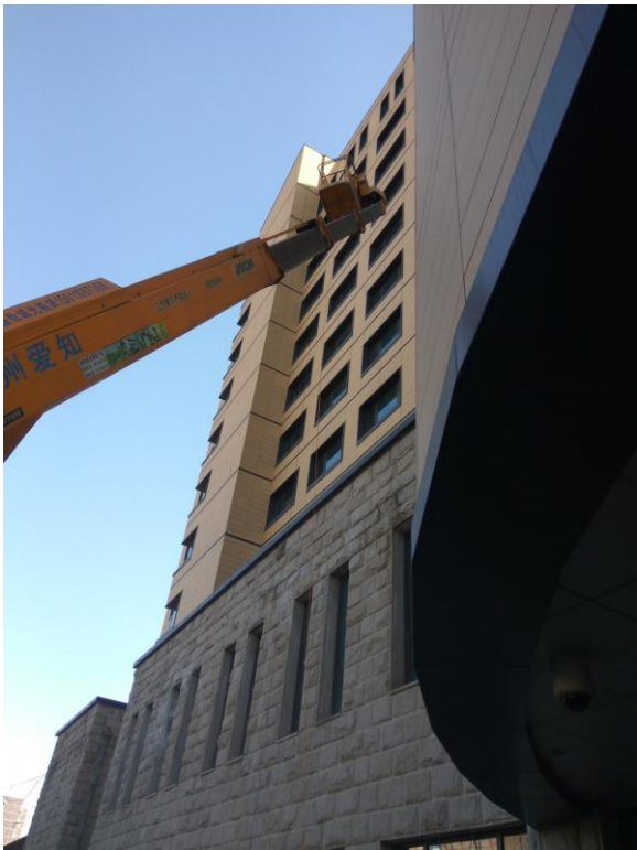
Typical measured point picture in building A
