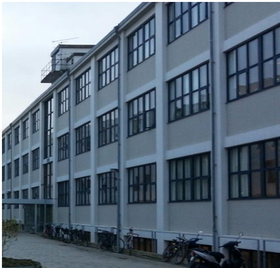
FIGURE 174 Traditional office building (STV)
