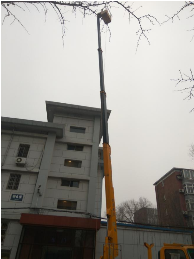
FIGURE 218 Typical measured point picture in building C
